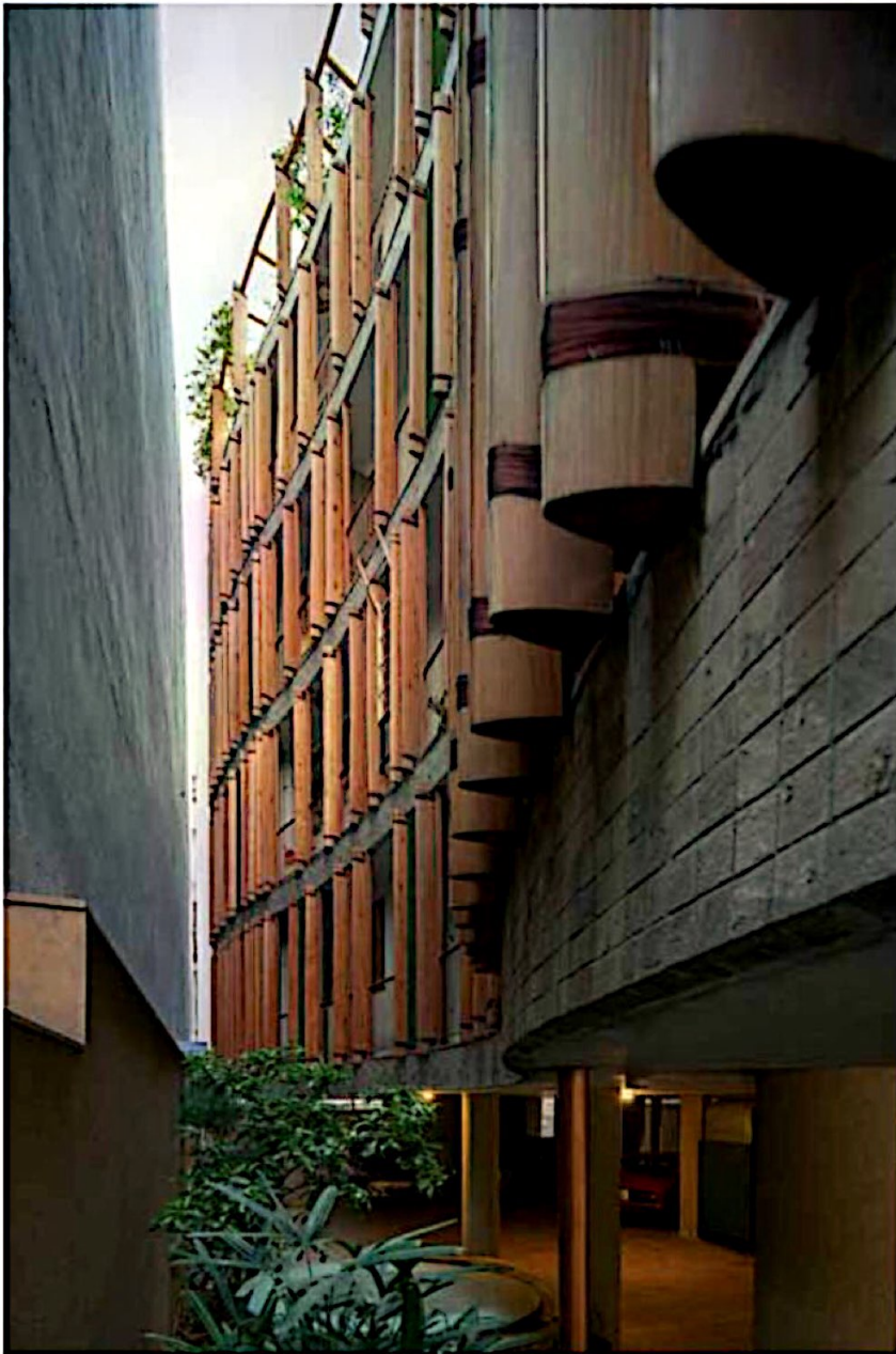
Below, left and right: comprising bespoke concrete formwork, the design of Outré House attempts to recentre the bond between making and material; bottom: a concept diagram showcasing the seamless façade that runs all along the building, providing sufficient ventilation and natural light
